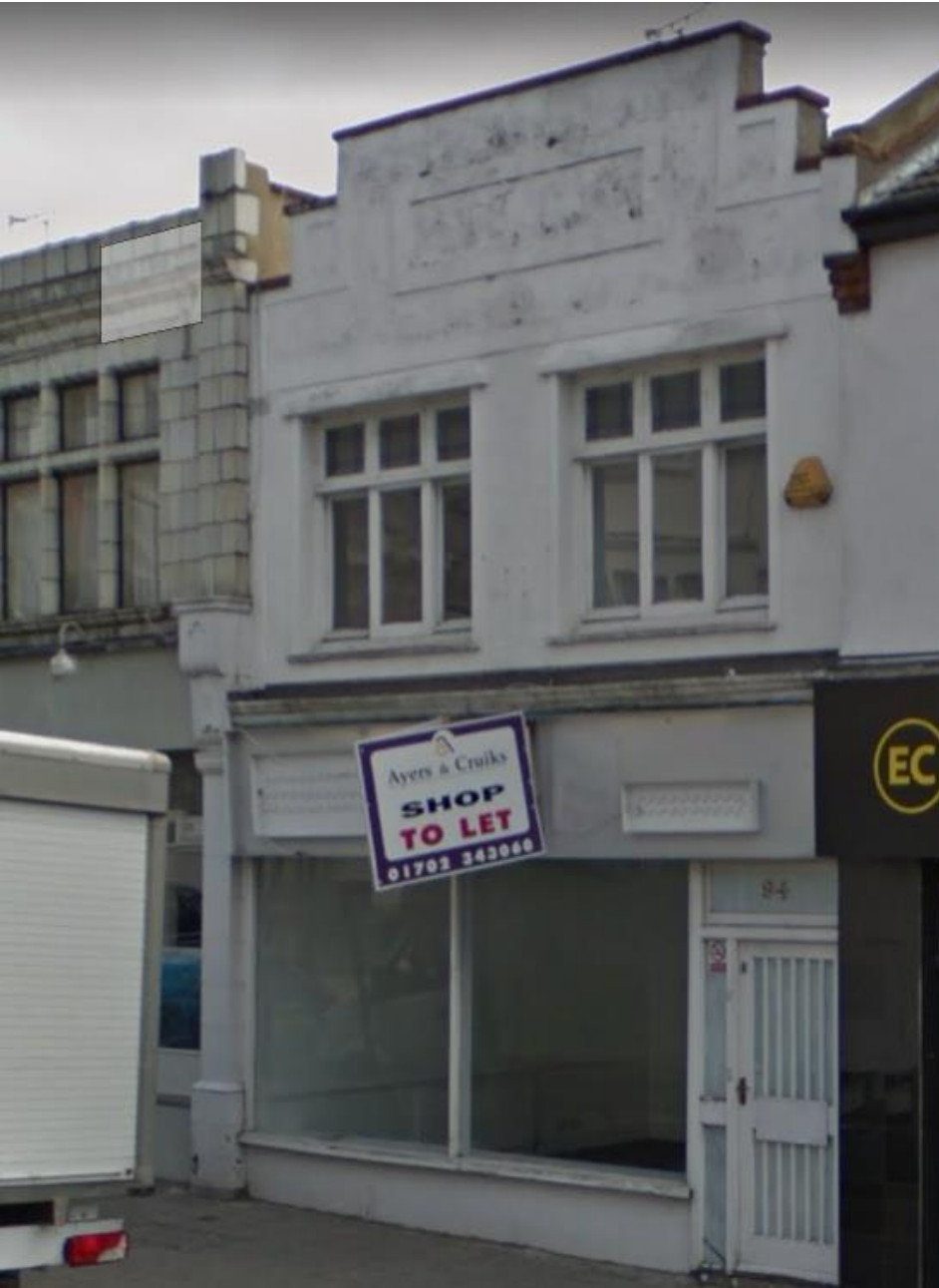
Timber shopfront and windows in 2018
